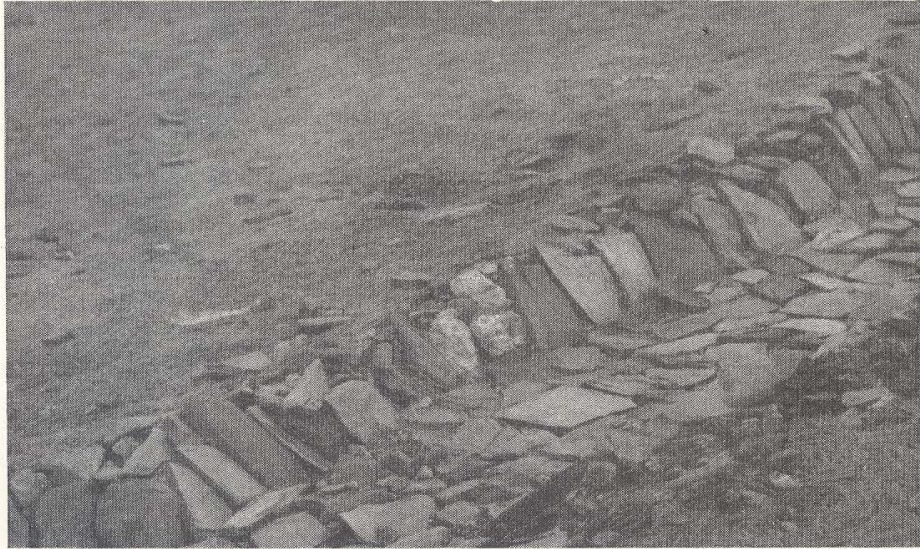
Figure 12.—The application of mulch and holding it down with netting is essential to provide suitable conditions for germination and establishment; paved drains are used for safe disposal of run-off
