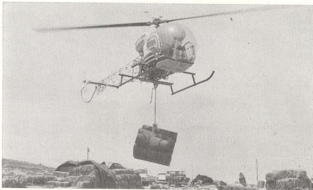
Figure 9. —Sling load of wire netting being transported by helicopter to Carruthers' Peak
