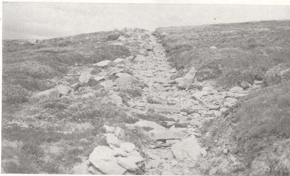
Figure 10. —Seriously gullied section of the Blue Lake track on the ridge down to Carruthers' Creek
