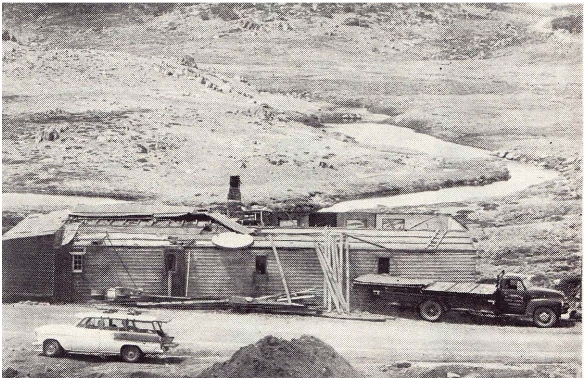
New Betts Camp being demolished in January 1963 (ASYB 1963)
