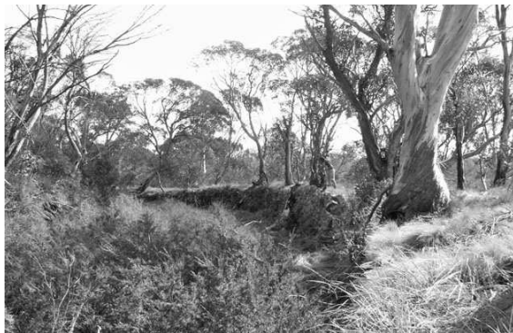
South Bloomfield Dam above Elaine Mine
