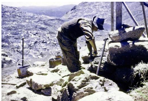
Granite foundation being built at Albina (Aust Alpine Club)
