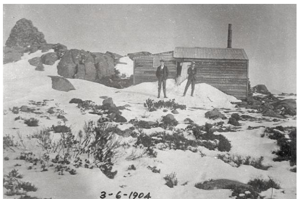
Fig 21. Mt Wellington Observatory Hut, sometime after its closure in 1898, J&M Grist Collection
