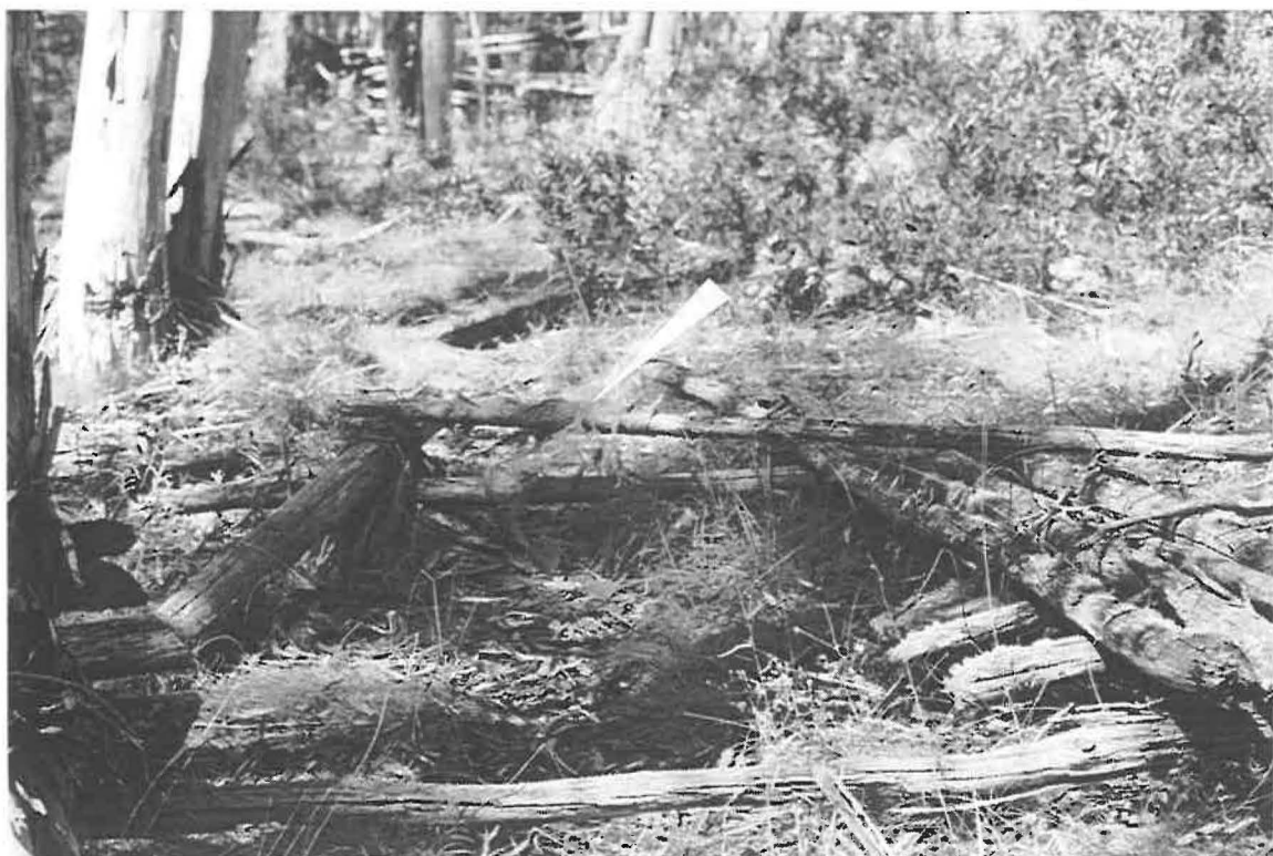
Photo 3, the collapsed northern entrance timbers; arrow points to remnant hessian.
