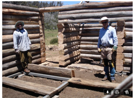
Simon Spinetti and Doug Pittard laying the floor slabs, photo KHA.
